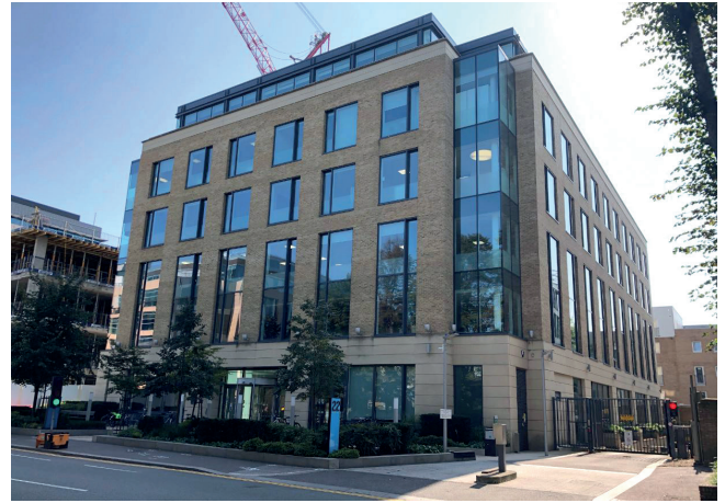
22 Station Road, Cambridge
