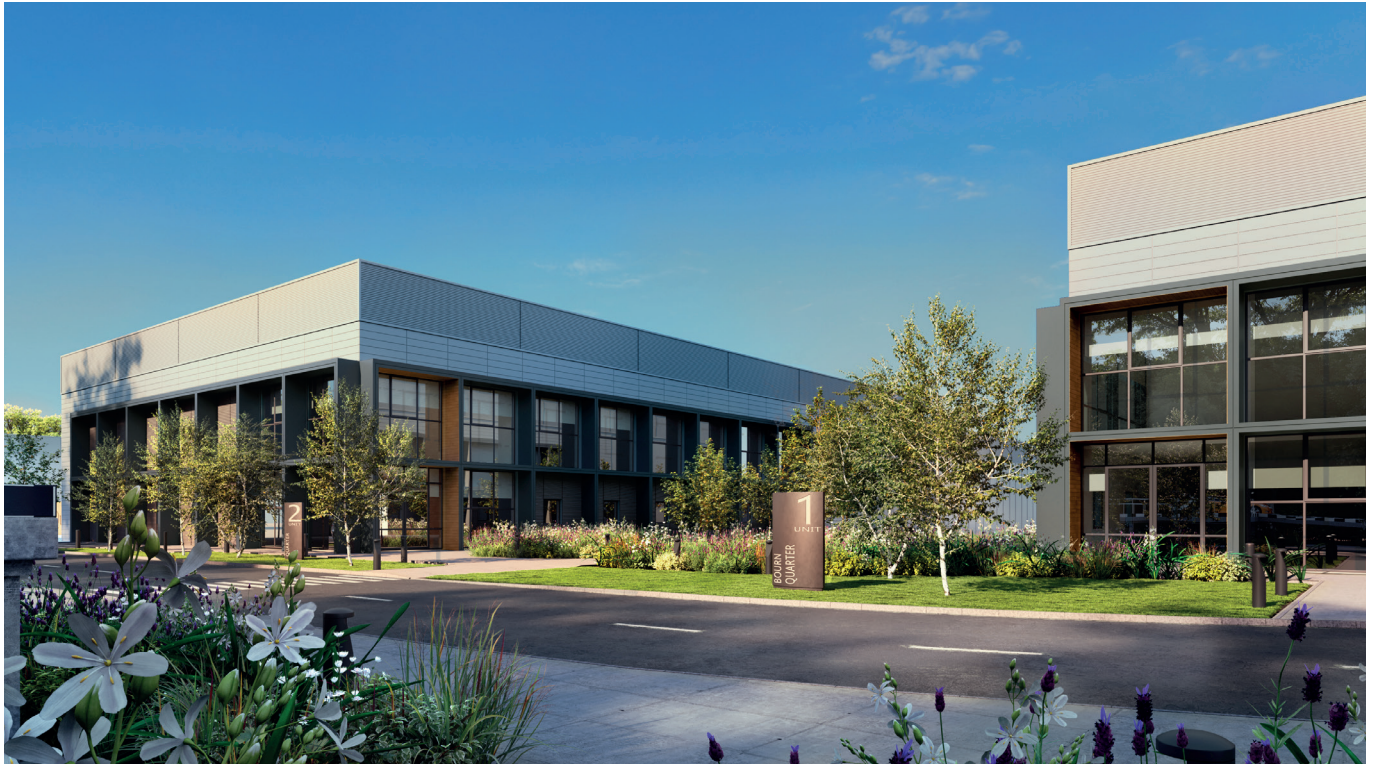
Bourn Quarter where over pre-lets have been secured on 80,000 sq ft of the 160,000 sq ft under construction
